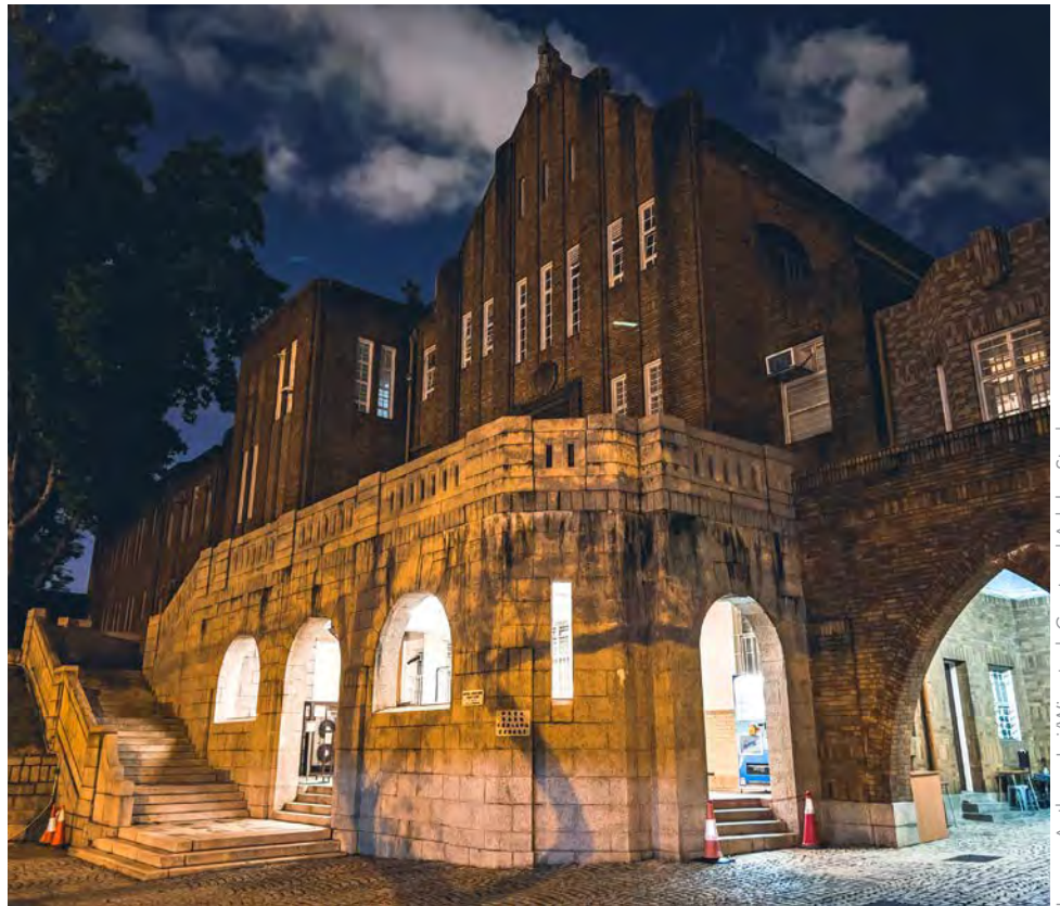
Maryknoll Convent School in Kowloon, Hong Kong at night
